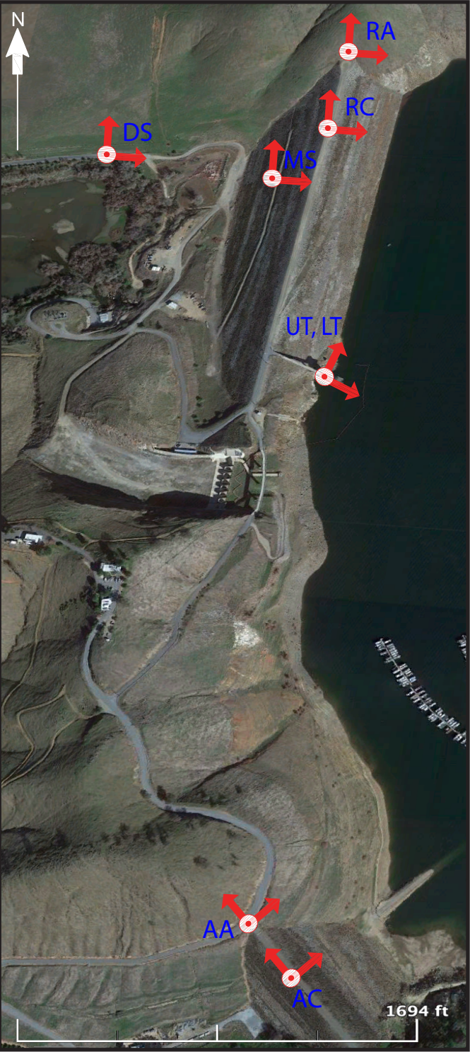
Main and Auxilliary Dam Area Overview
